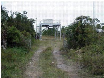
Storm hardening requirements are considered in the engineering and design process. This elevated cabinet, positioned on coastal terrain, was built 20 feet in the air to avoid storm surge.
